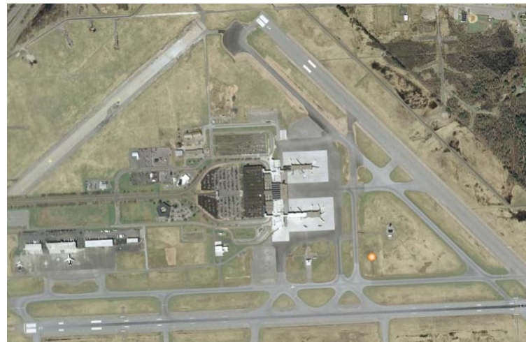
Hancock Airport- From Google Earth
